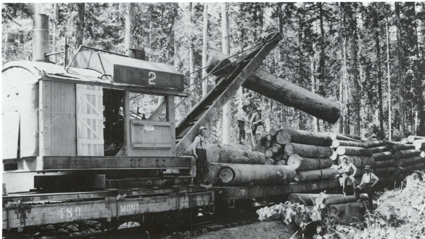
ABOVE: Logs were loaded by a Marrison Loader on flat cars to be hauled to the mill. BELOW: Housing for the crews was frequently moved and set up as home for the lumberjacks.
