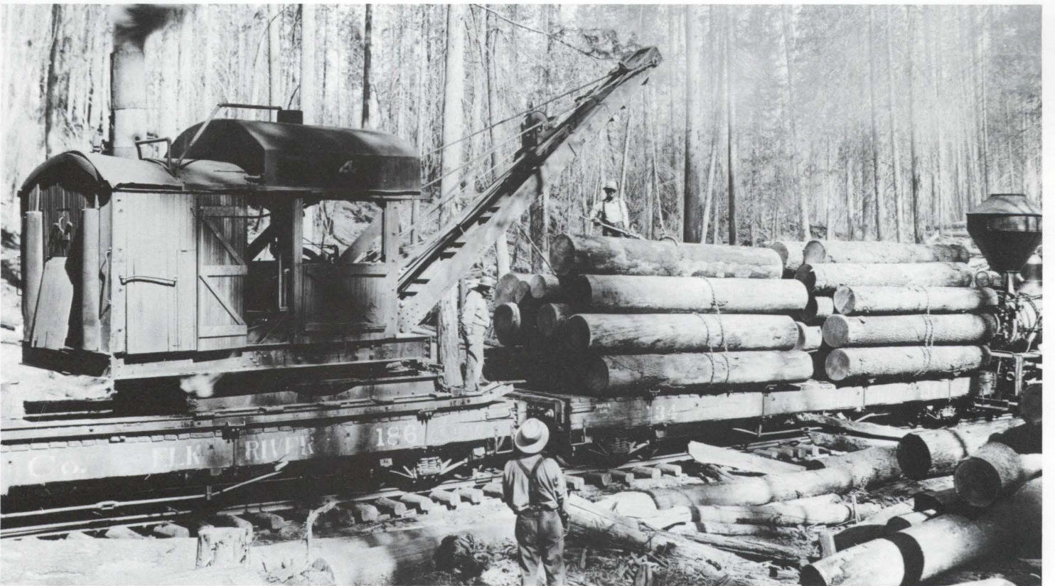
ABOVE: Chaining the logs together to be pulled out on a dolly by teams of horses. BELOW: A Marrison loader with loaded flat cars and engine in the background.
