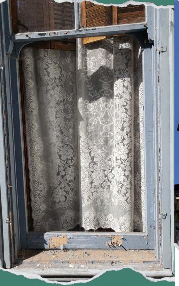
The Mansion has 41 windows, all with their original panes of glass. As you can see in the photos, the paint around the glass is weathered and exposing the underlying wood. Without addressing these issues, the wood will continue to deteriorate, compromising the surrounding structure. Animal activity has damaged some of the eaves on the second floor, which would also be repaired.
