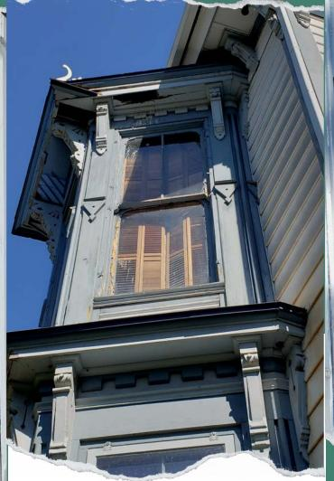
These problems require skilled woodwork to salvage existing materials, replace rotted wood, paint, structurally repair the areas around the windows and interior window sills, and install permanent storm windows.
