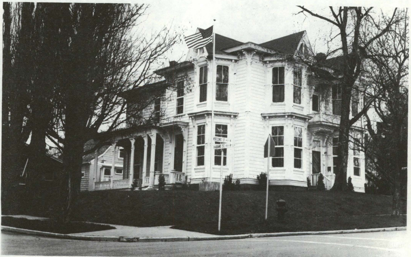
Mansion before 3-color paint and restorative work on south balcony. LCHS photo.
