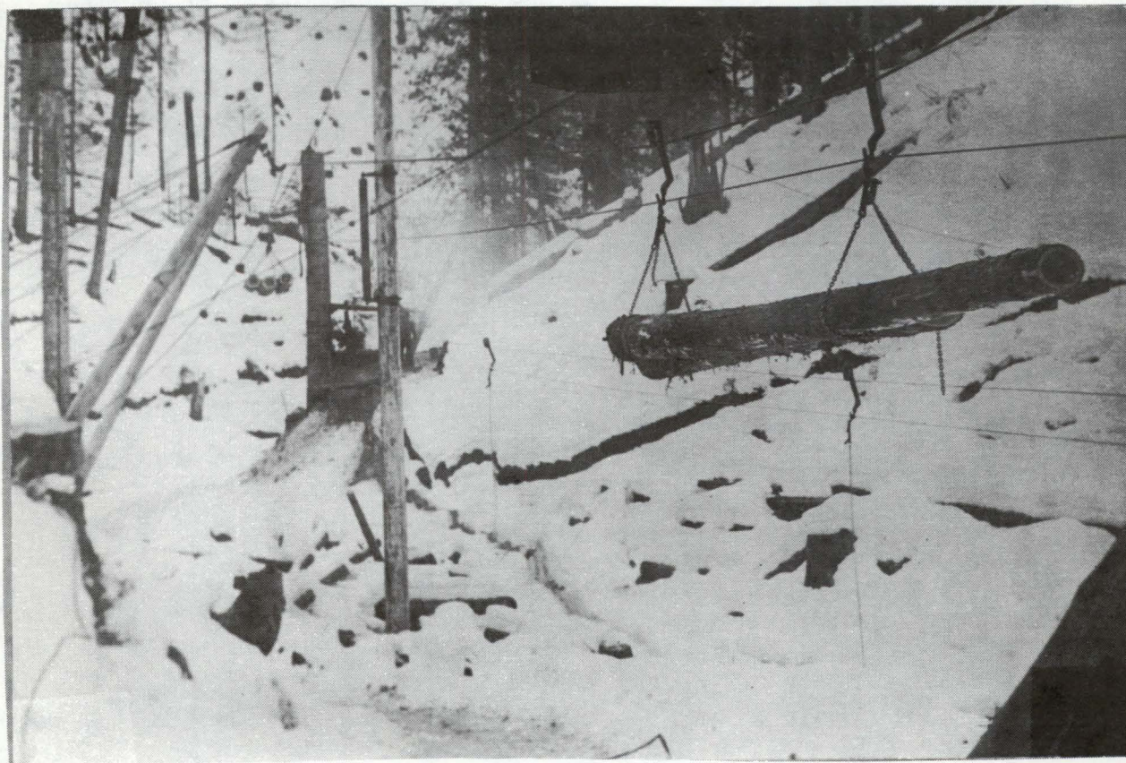
Highline Logging, with Donkey Engine
